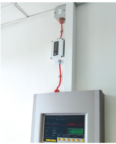
Figure 2: Installation of ready-boxed ESP Protector outside the equipment panel on a fused connection of 5 A or less (ESP 120-5A/BX, ESP 240-5A/BX, ESP 277-5A/BX) or 16 A or less (ESP 120-16A/BX, ESP 240-16A/BX, ESP 277-16A/BX).
