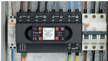
Figure 1 - ESP 415 D1/LCD installed on a DIN rail within a power distribution panel.
