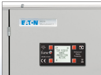
Figure 5 - ESP 415 D1R/LCD remote display installed on the front of a power distribution panel.
