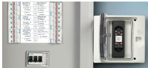
Figure 2 - ESP 415 D1/LCD installed next to a power distribution panel in a suitable WBX D enclosure.
